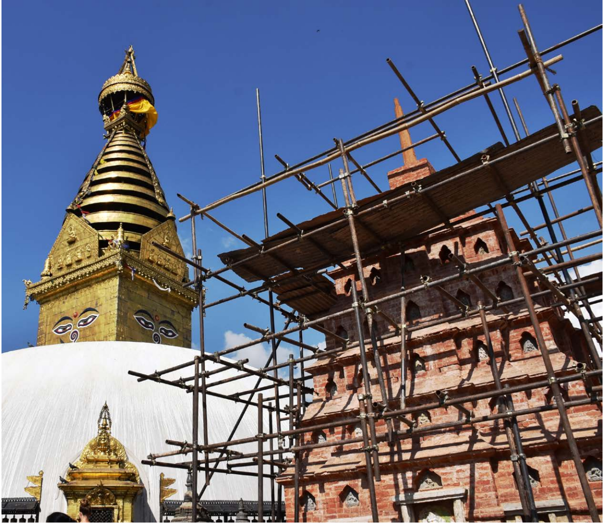
Restoration of Tashi Gomang Stupa (Mangal Bahudwar Caitya) at Swayambhu. © UNESCO
