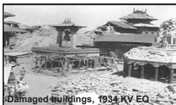
Damaged buildings, 1934 KV EQ
