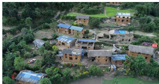
Earthquake affected houses of Triveni, Ward 1, Nalgad Municipality, Jajarkot. Picture courtesy of UNDP Nepal
