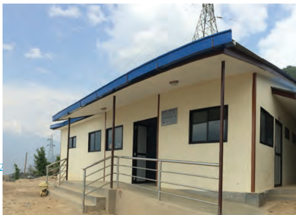
Building of a health facility reconstructed after earthquake
